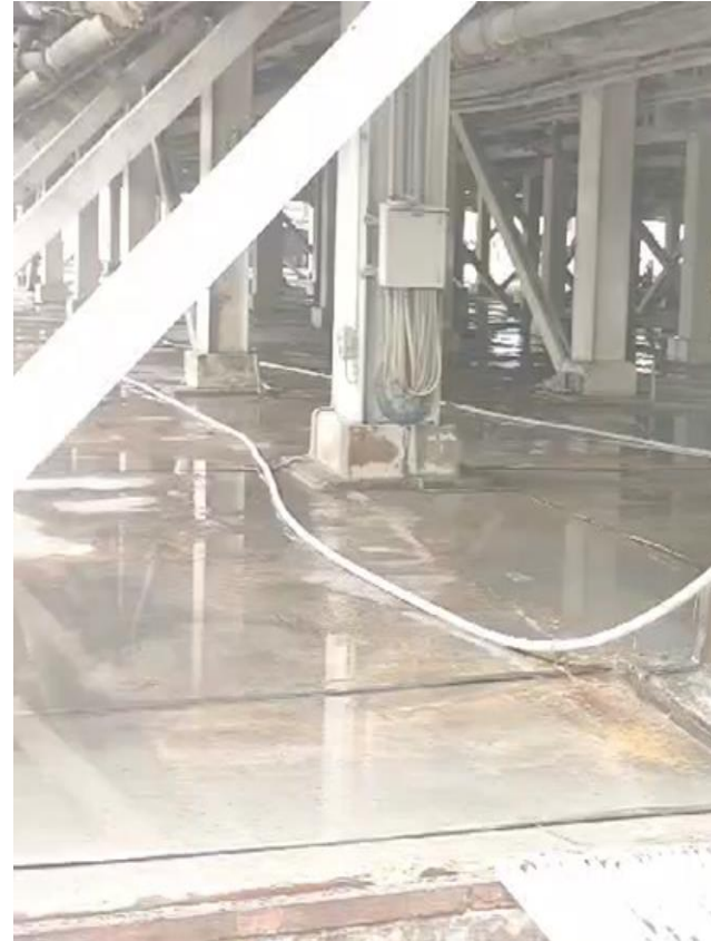
Cleaning of ESP Area by using ETP Water.
