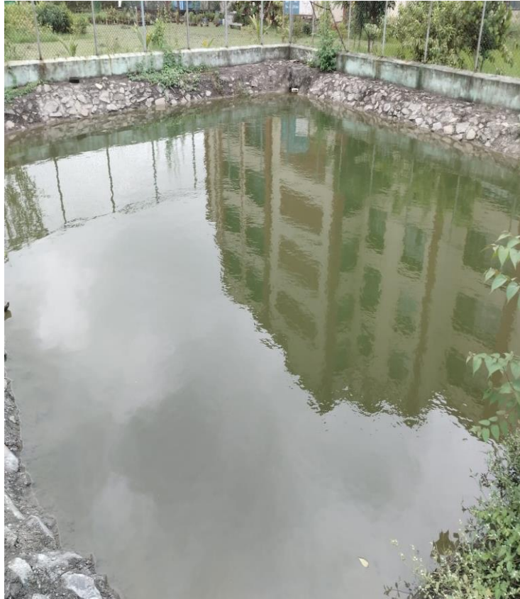
Roof Rainwater Harvesting System
