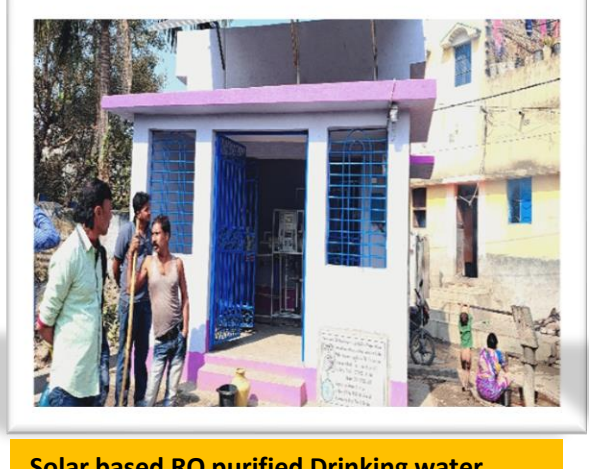
Solar based RO purified Drinking water system at Diarrhea prone village
